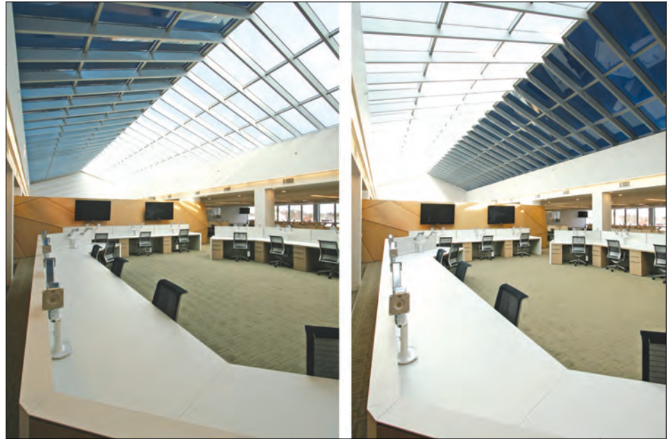
Windows with electrochromic glass can be tinted in minutes with the push of a button. This building in Greenwich, Conn., shows how different windows can be tinted at different times.
