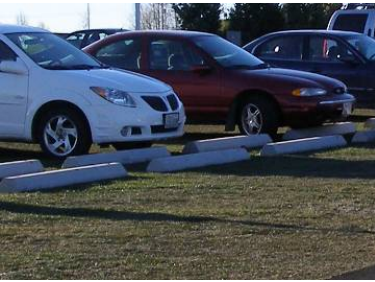
Unmanaged stormwater can lead to severe erosion (top).
